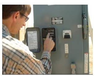
Figure 2. Clock timer used to automatically shut a groundwater well off before 12pm and turn it back on after 6pm every weekday during the peak season.
